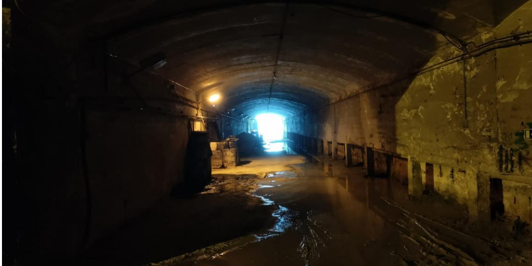
Figure 7: Access tunnel to the A-Station from Triq Fra Diegu in Marsa (photo dated 2023).
