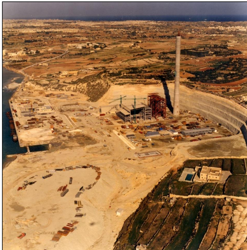
Figure 2: Delimara Power Station during the initial phases still under construction.
